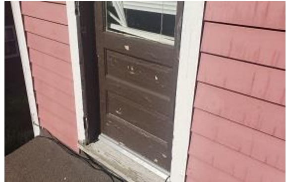
Door and components B (2 nd floor)
