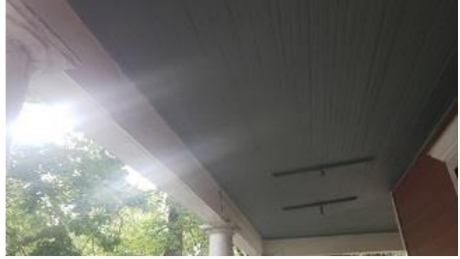
Porch A porch ceiling and porch beam
