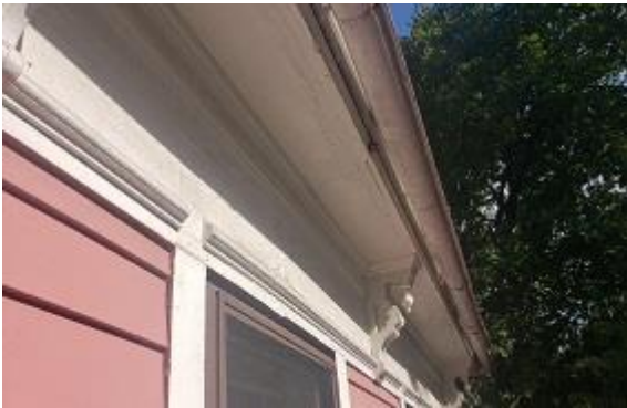
Soffit, fascia, and frieze board ABCD
