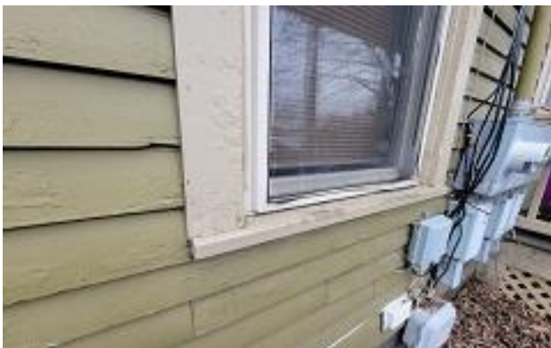
Siding, window casing, and sill C
