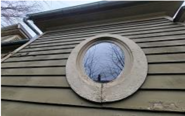
Window and casing B
