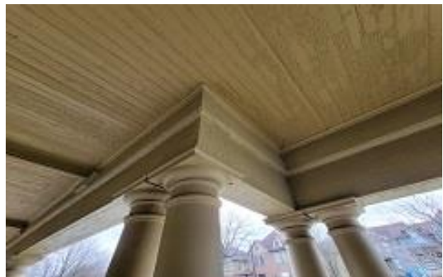
Porch A support beam
