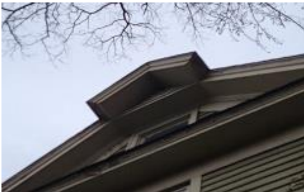
Attic window and casing, upper Trim, soffit, and fascia D (assumed positive)
