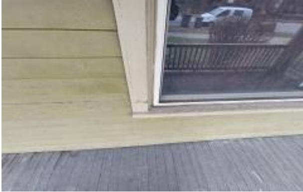
Window casing, sill, and siding ABCD
