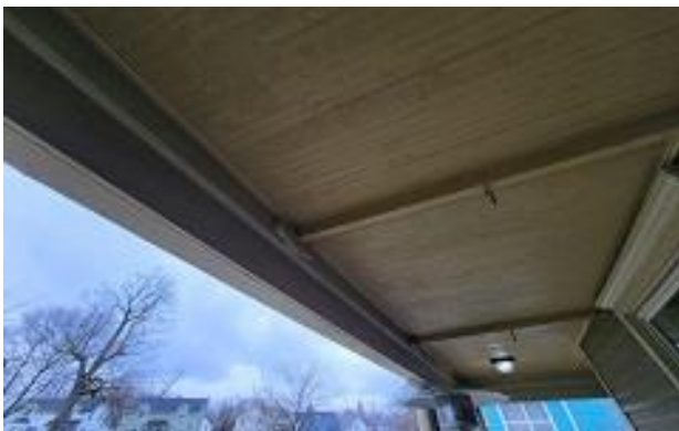
Porch A ceiling
