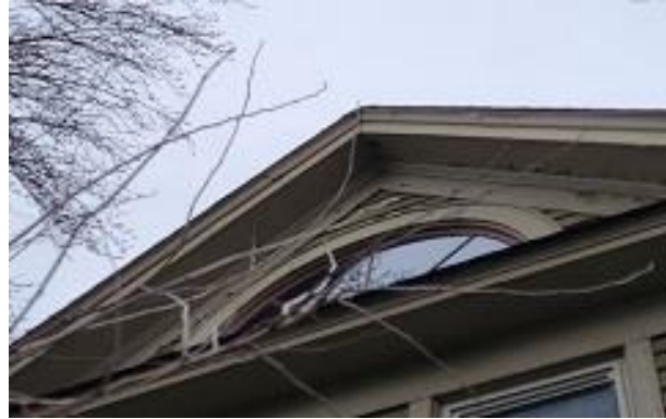
Attic window and casing, soffit, fascia, and upper trim B (assumed positive)
